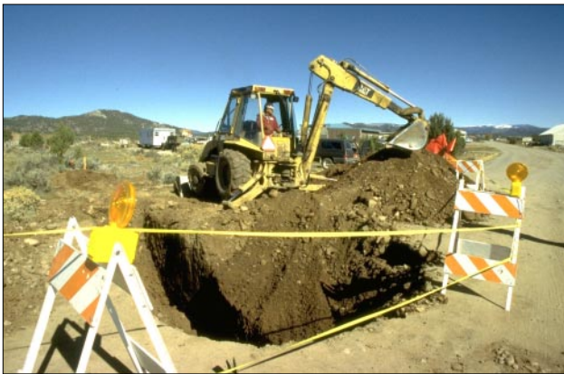
Figure 5. Photograph of backhoe removing road gravel and upper structure fill.
